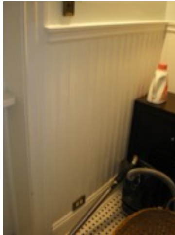
Work areas and former servant spaces in the Willock House would likely have contained vertical, tongue-and-groove, wood wainscoting like that seen in a third floor bathroom at the Childs House (above left) and a back bathroom on the second floor (above right).
