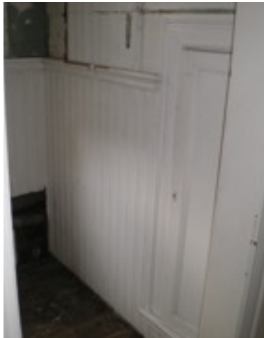
Work areas and former servant spaces in the Willock House would likely have contained vertical, tongue-and-groove, wood wainscoting like that seen in a third floor bathroom at the Childs House (above left) and a back bathroom on the second floor (above right).
