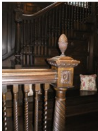
While more ornate than at the Willock House, the balustrade at the Childs House illustrates Proctor's attention to detail and repeated use of carved rope twist balusters.
