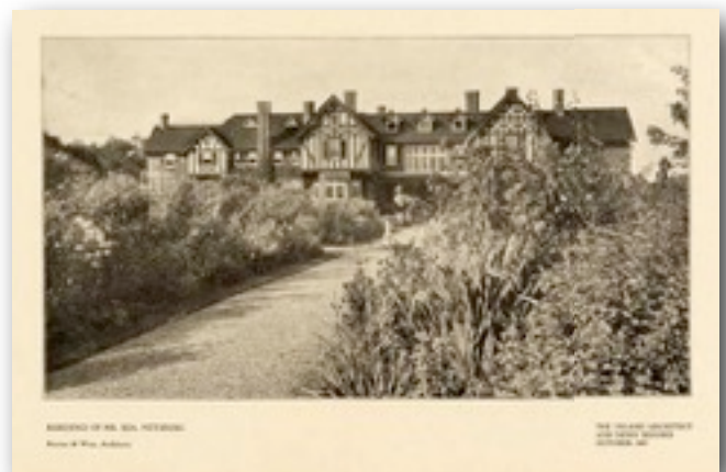
Henry Rea Residence, Sewickley Heights, 1900 ( Inland Architect and News Record ).
