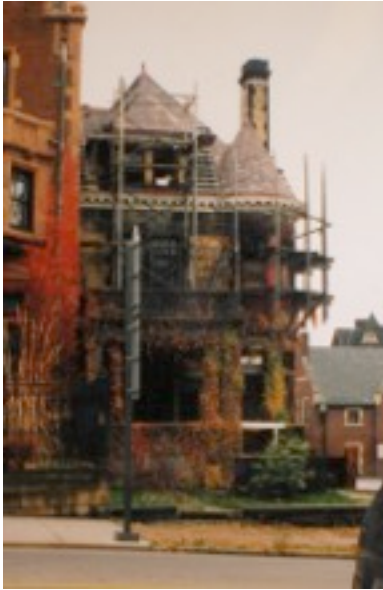
Scaffolding erected during the Costa's ownership.
