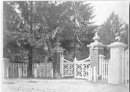
Entrance Gates at Sewickley, PA, William Ross proctor, Architect, H.L. Wass, Associate (Pittsburgh Architectural Club, Catalogue of the Annual Exhibition, 1900 ).
